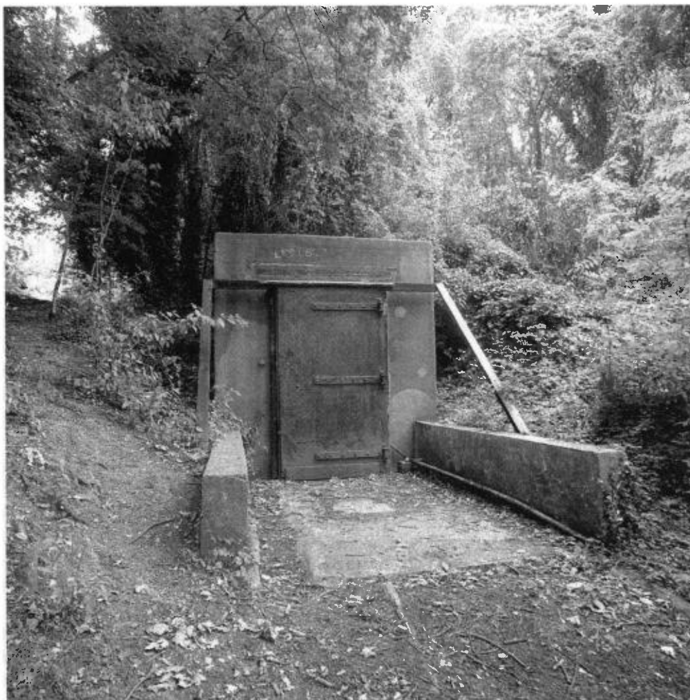
The emergency exit
